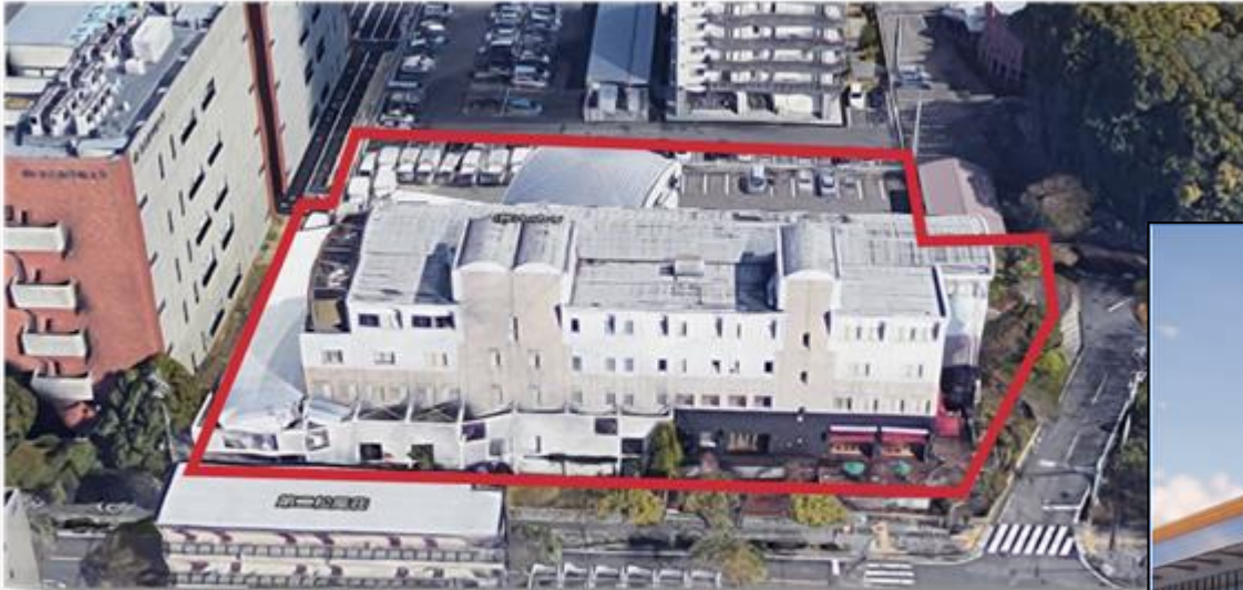
Nagoya, Japan, distribution facility
